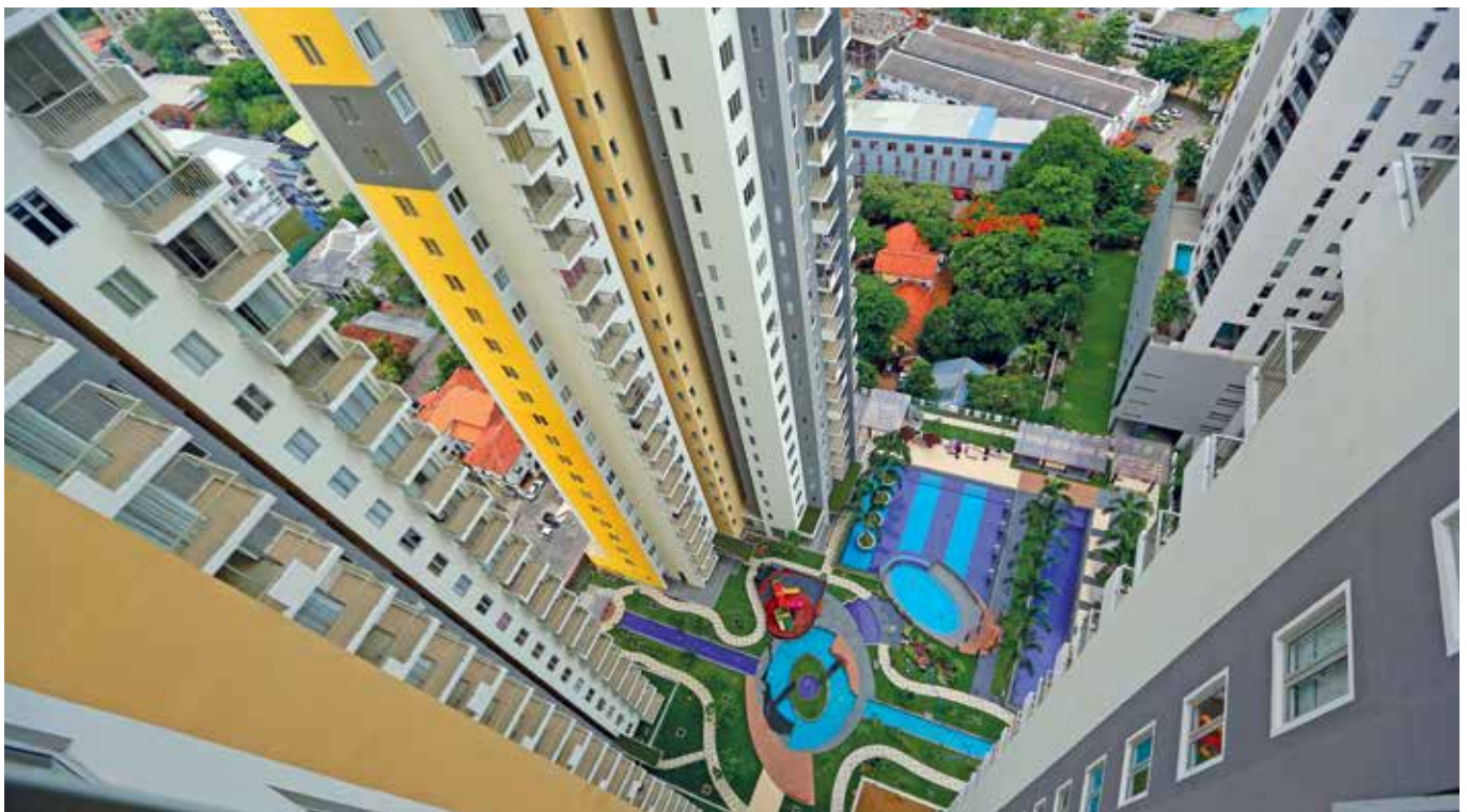
The construction of the "OnThree20" residential development was completed on schedule
